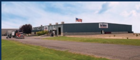
Bridon USA Twine factory in Jerome, Idaho
