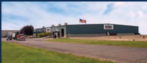
Bridon USA Twine factory in Jerome, Idaho
